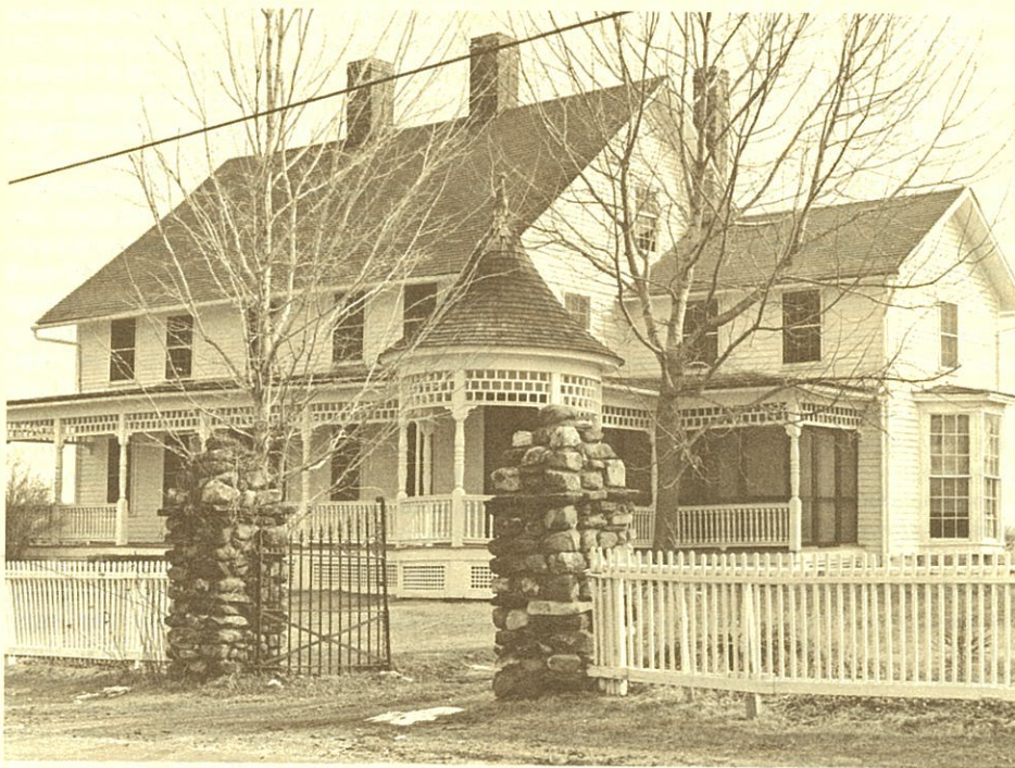
Figure 3. Later Georgian Farmhouse of the Second Phase of Settlement, southern section of East Street. Diagnostic features include the symmetrical facade, five bays, and double chimney. The front porch is a marvelous example of a Victorian veranda. Note the bay window on the addition to the right. This double chimney style of Georgian architecture was popular all over Goshen between the Revolution and 1820.
