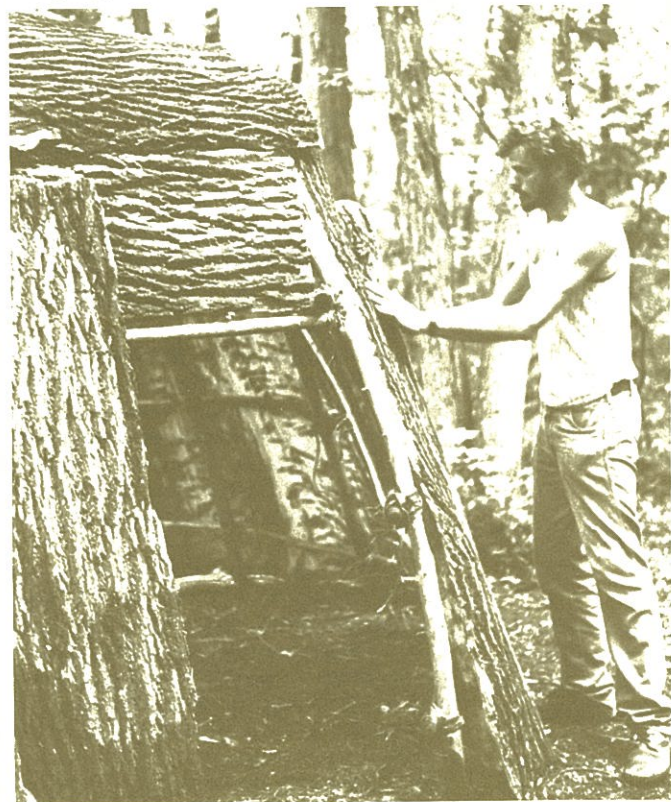
2. Jeff Kalin fitting bark to wigwam frame
